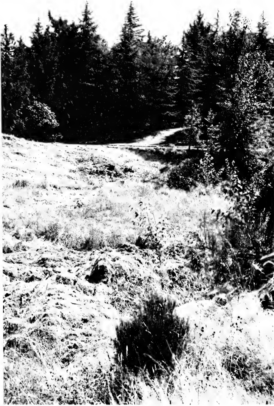
Conifer Meadow area before the beginning of construction, August 1980. Photo: J.A. Witt
